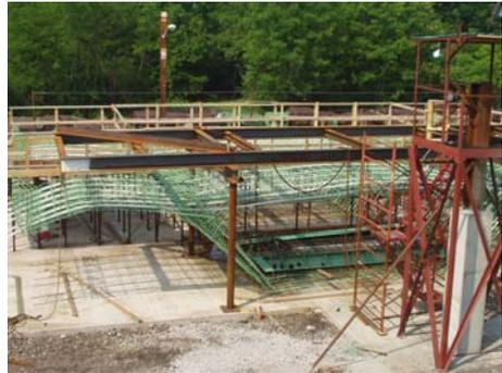
The Susquehanna Segmental Bridge on the Pennsylvania Turnpike is currently under construction. This bridge is the first major bridge in Pennsylvania to utilize post-tensioned segmental construction. Precast, post-tensioned segmental bridges have the advantage of excellent durability and long service life combined with quick
