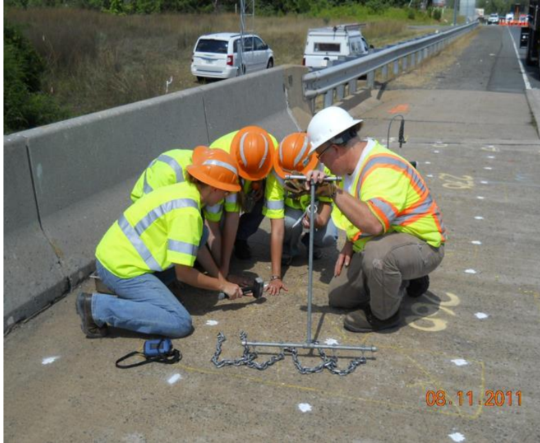
Figure 94. Inspectors conducting chain drag on deck. (FHWA 2013)
