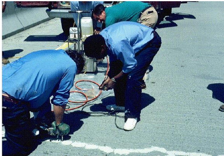
Figure 31. Epoxy Injection Procedure (VirginiaDOT 2009)
