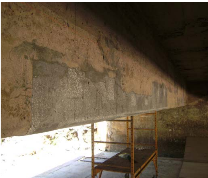
Figure 7: Beam 4 after Patch Repair
