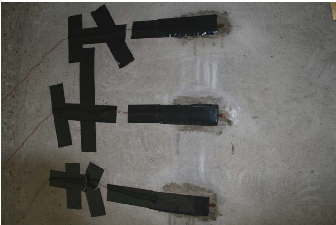
Figure 42: Concrete Gages with Barrier E Protective Coating
