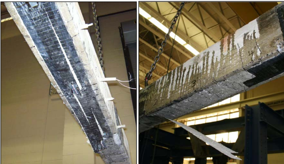
Figure 118: Photos of fatigued Part II beams repaired using Wrapping Scheme 2 after failure
