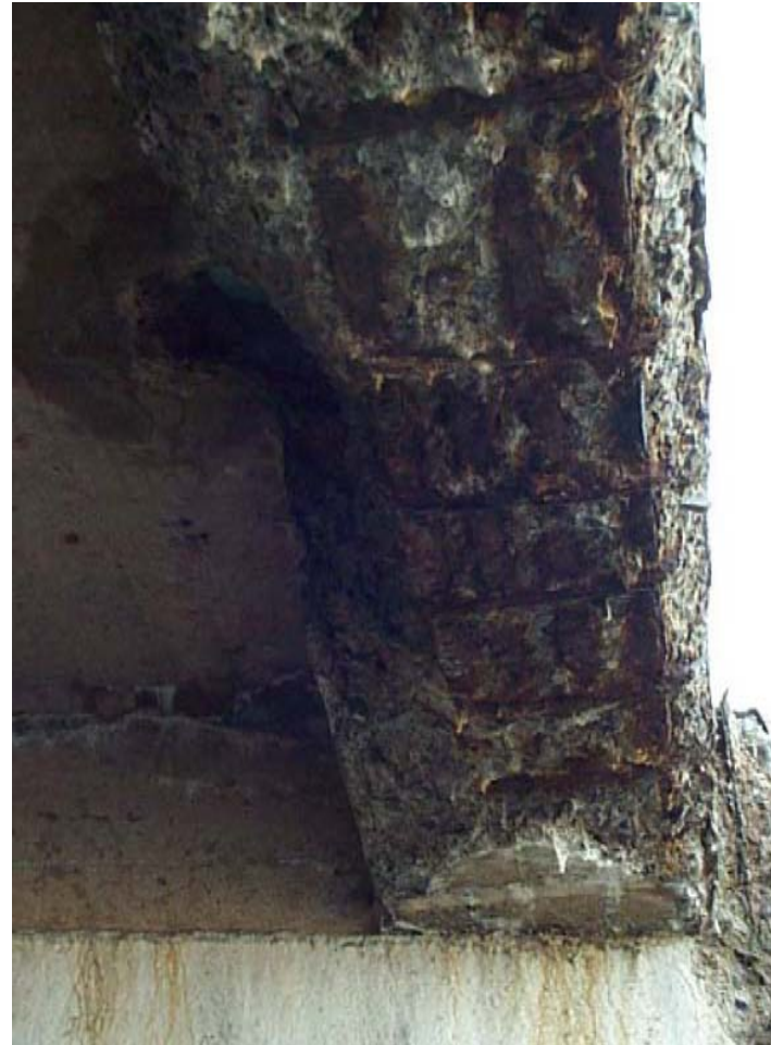
Note: This is a likely candidate for repair. This bridge scored high because of its high traffic volume and similarities in damage to the NCHRP Report 514. This bridge ranked high even though it scored relatively low in the span and age categories.
