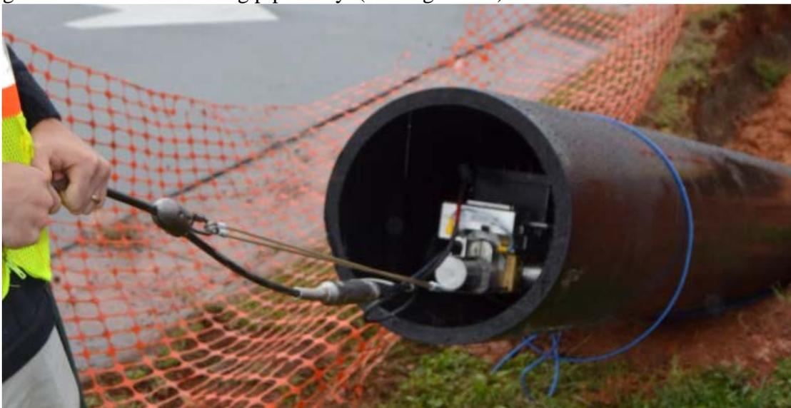
**Figure 19. FutureScan Robot being inserted into Utility at Burnt Chimney Site (Photo by Lindsay Ivey Burden).**
