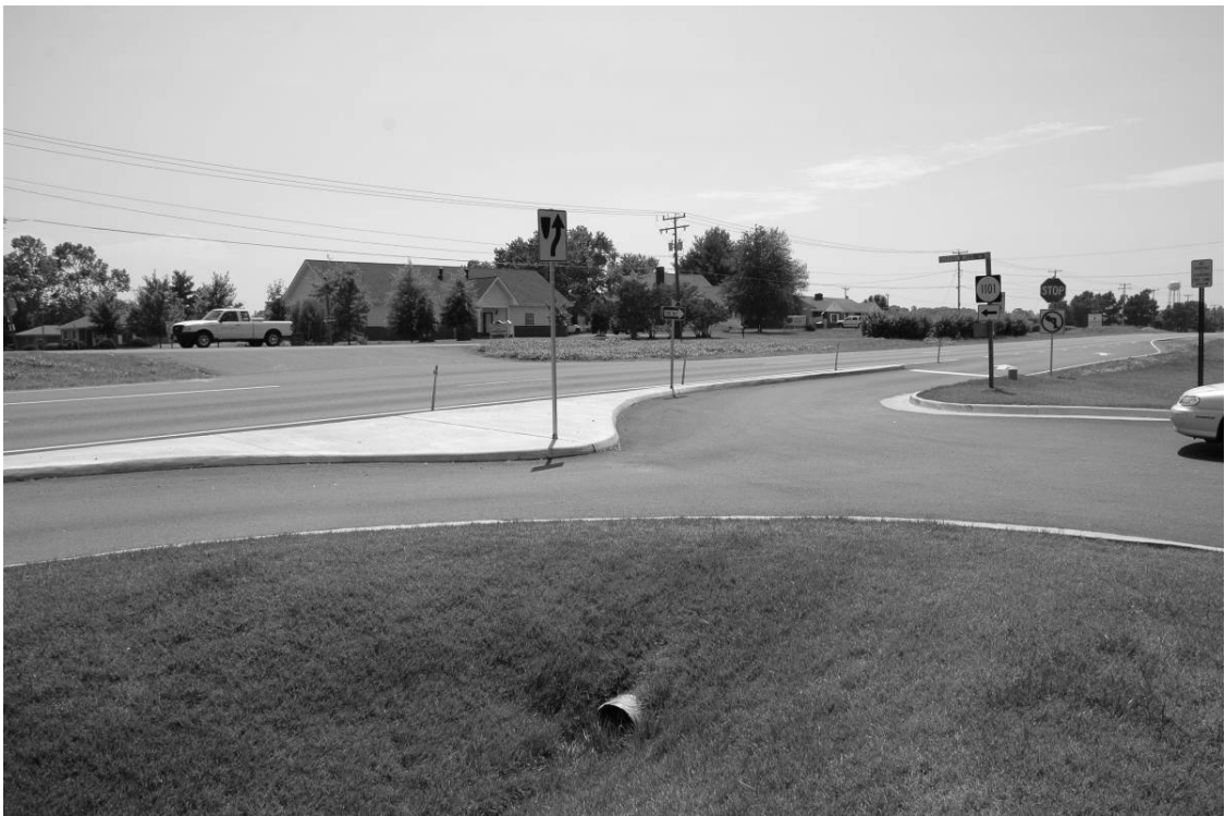
Figure 1.2.1: Intersection with turning movements restricted. The island at this driveway restricts left turns, thus reducing the number of conflict points. Intersection with westbound Route 3, across from intersection with Route 1101 (Sheraton Hills Drive), Spotsylvania County. Photograph by author.
