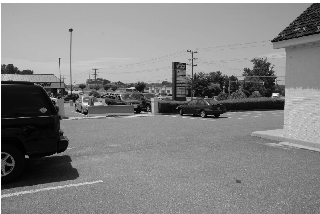
Figure 1.2.4: Restricted access between two parking lots. The concrete barrier in this photograph blocks access between the parking lots. This forces vehicles back onto the main roadway to travel between the properties. Southern side of Route 3, looking towards signal at intersection with Route 694 (Heatherstone Drive), Spotsylvania County. Photograph by author.
