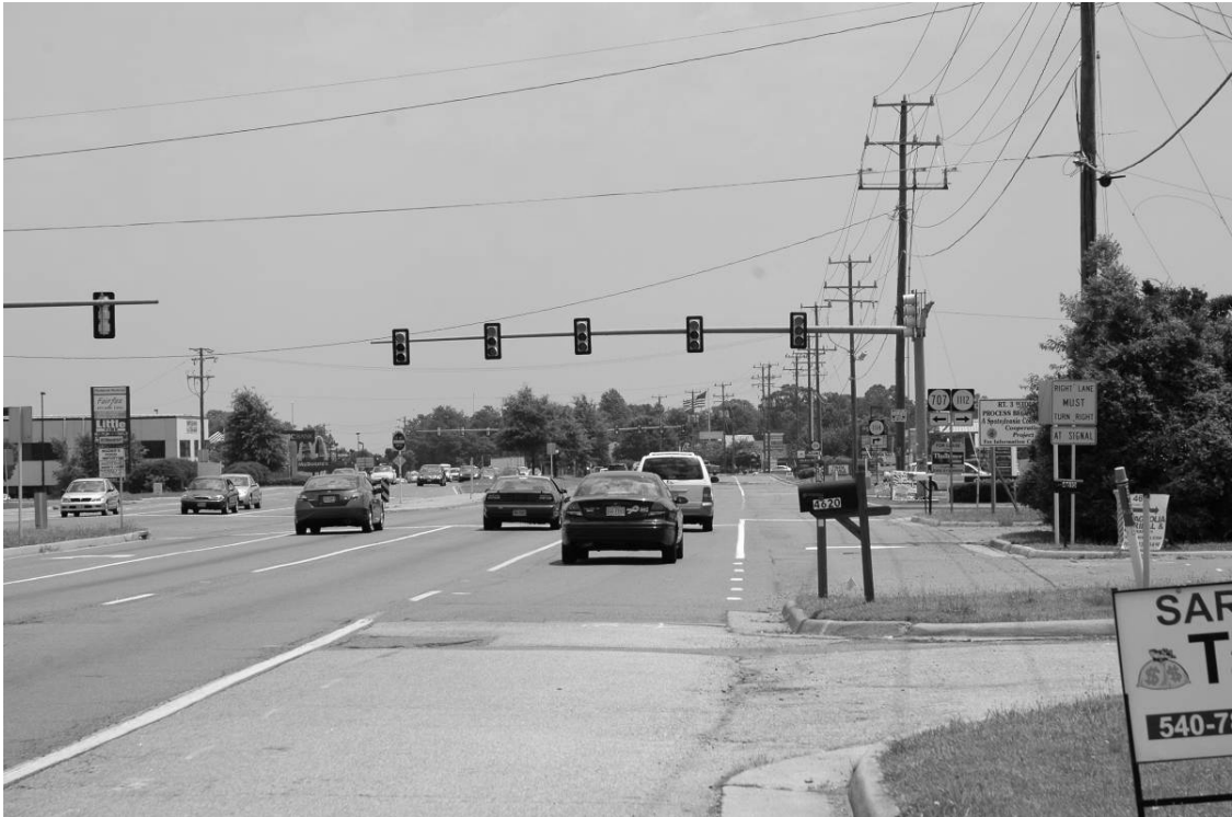
Figure 1.2.3: Numerous closely spaced driveways create a confusing situation for drivers. Eastbound Route 3, looking at intersection with Routes 707 and 1112 (Chewing Lane and Rutherford Drive), Spotsylvania County. Photograph by author.
