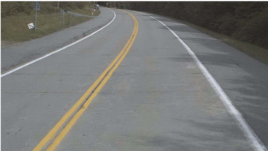
Figure 4. Example of Pavement Score = 7 in New York State (NYSDOT, 2010).
