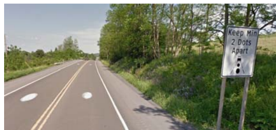
Figure 27. Example of aggressive driving “dots” sign and pavement markings.
