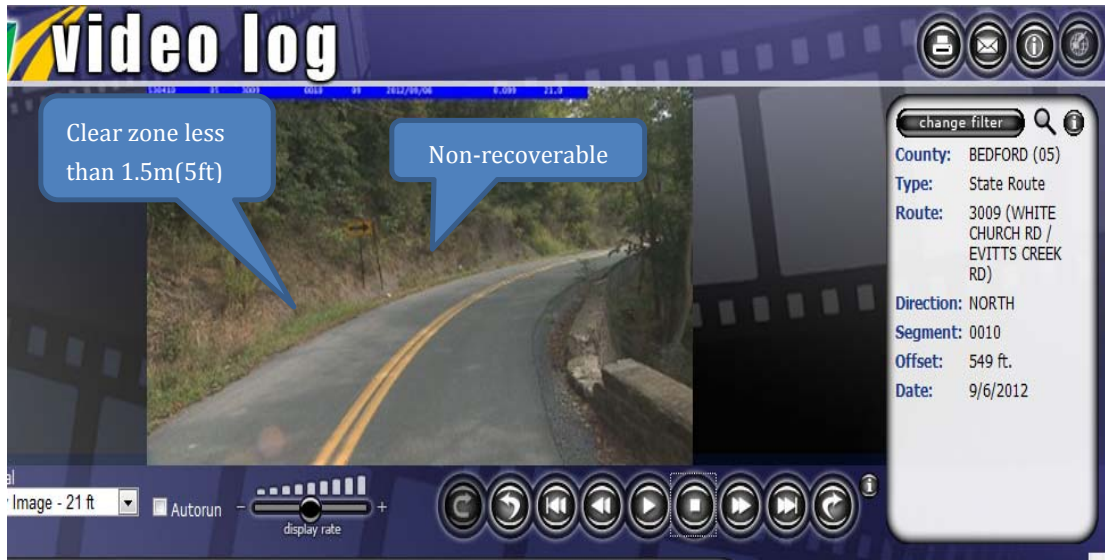
Figure 18. Video Log for SR 3009, Segment 0010.
