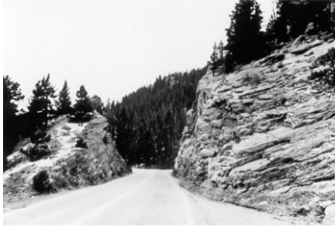
Figure 17. Roadway with Roadside Hazard Rating Equal to 7.
