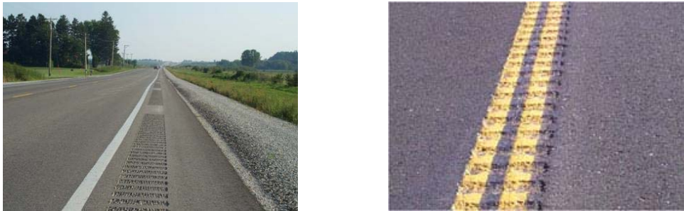
Figure 25. Example of centerline rumble strips (left panel) and shoulder rumble strips (right panel).
