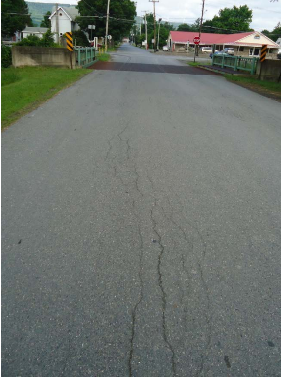
(a) Eastbound Lane Longitudinal Cracks
