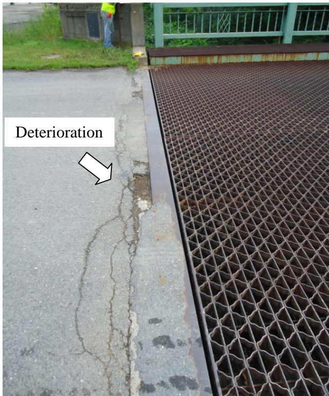
(a) West Transition Pavement Damage
