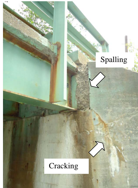
(b) Cracking and Spalling
