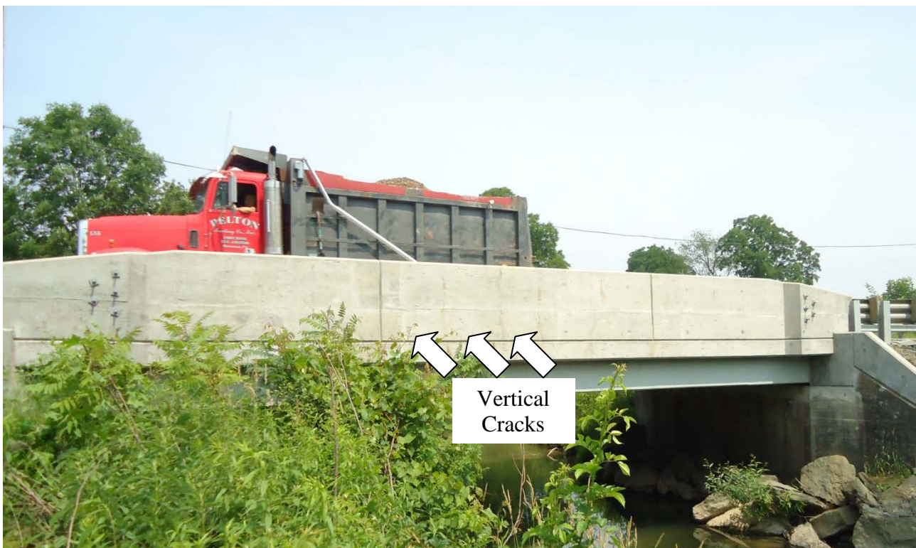
Figure 11. Bridge Four Elevation
