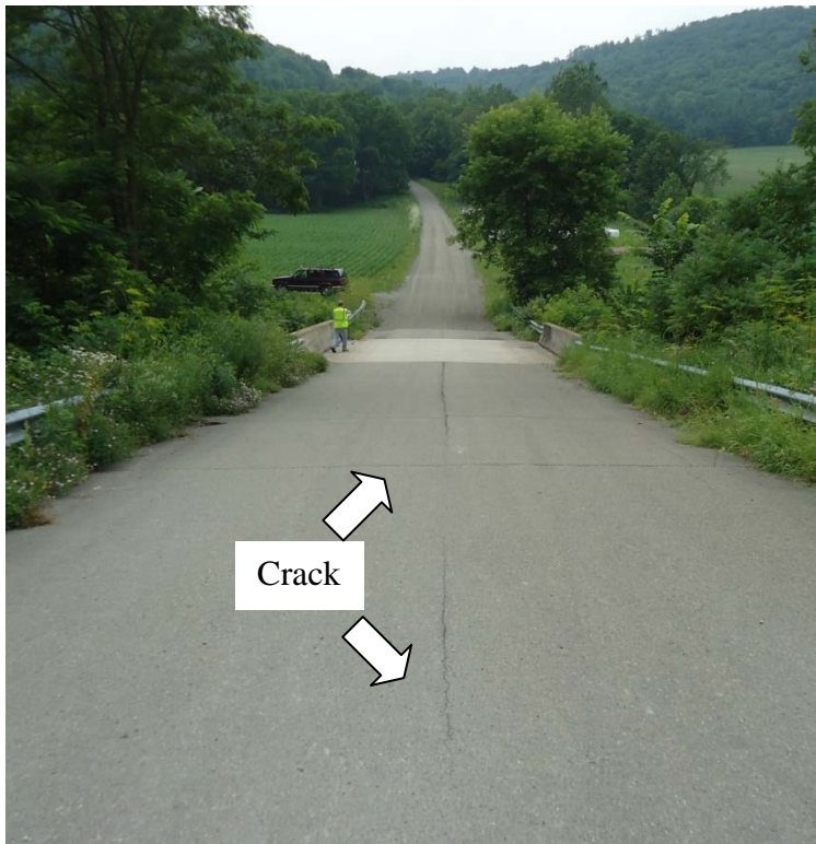
(a) Longitudinal and Transverse Cracks
