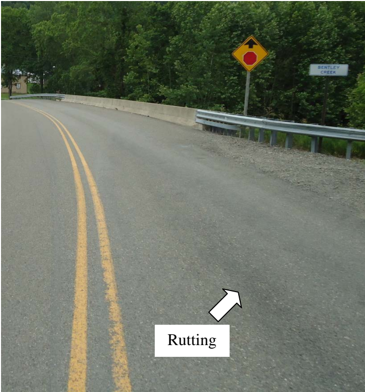
(a) Eastbound Lane Rutting
