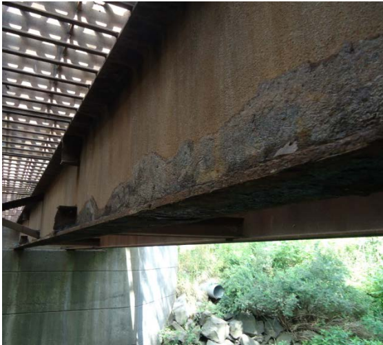
(a) Beam Ten Corrosion
