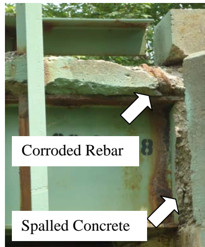
(b) Spalled Concrete and Exposed Rebar
