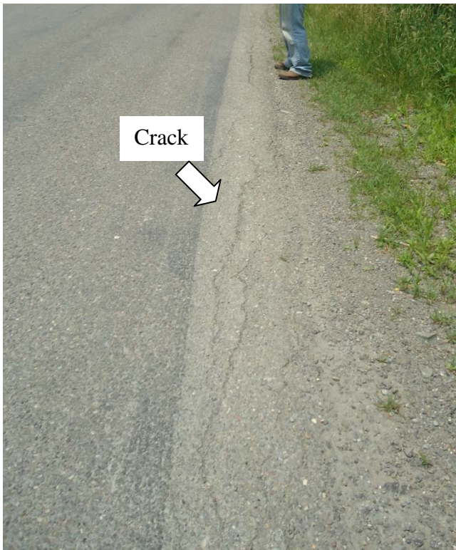
(a) Shoulder Longitudinal Cracking
