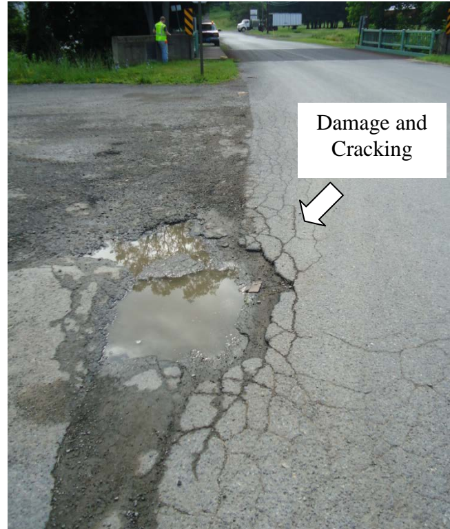
(b) Westbound Lane Edge Pavement Damage and Cracking
