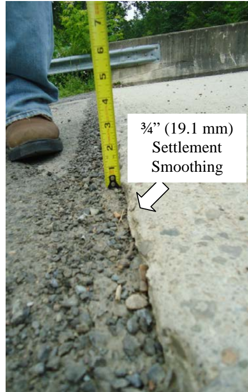
(b) Settlement above South Abutment
