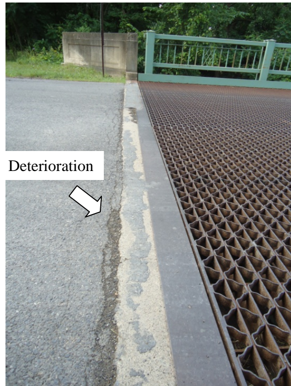
(b) East Transition Pavement Damage
