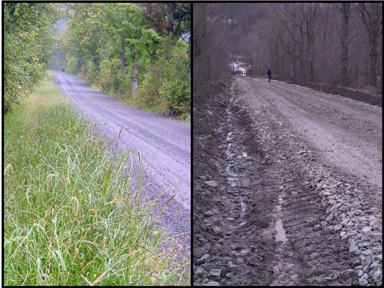
Figure 36a,b. Side by Side Comparison of a Well-Implemented Gravel Road [a] before the Heavy Gas Truck Traffic and [b] after Exposure to the Heavy Traffic
