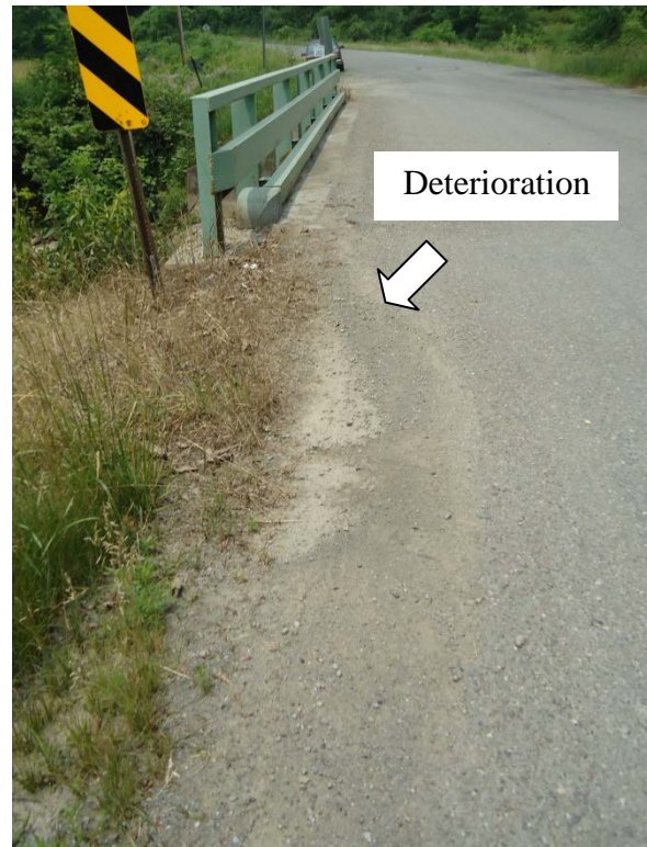
(b) Pavement Deterioration at Bridge Transition
