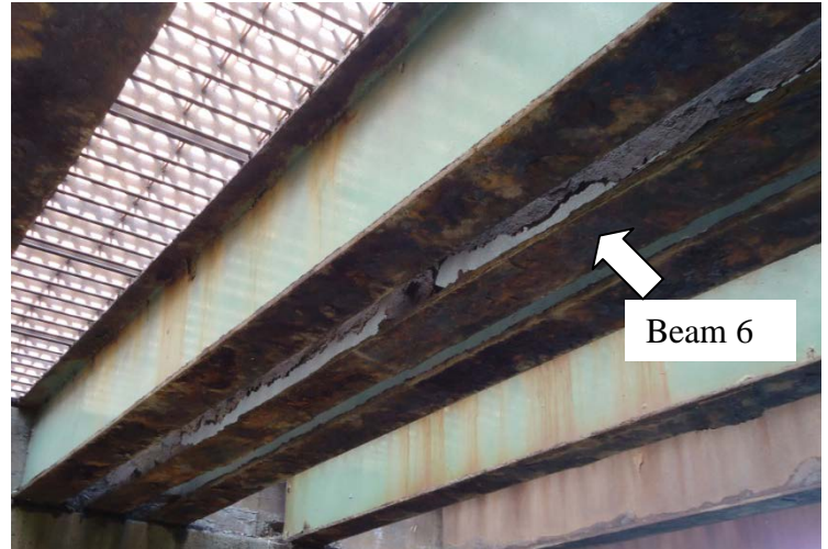
(b) Beam Six Corrosion and Section Loss
