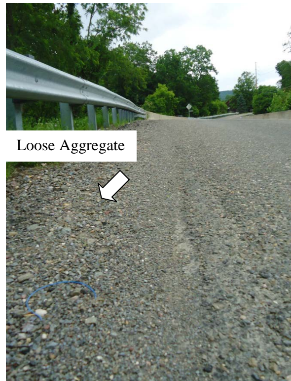
(b) Shoulder Loose Aggregate
