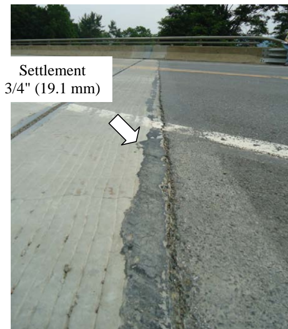
Figure 15. Bridge Five Settlement at South Abutment
