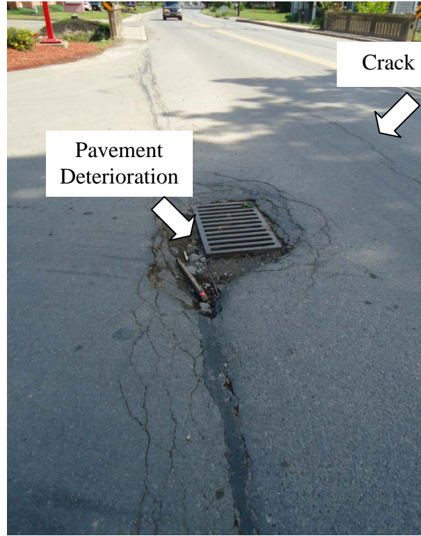
(b) Pavement Deterioration and Longitudinal Cracks
