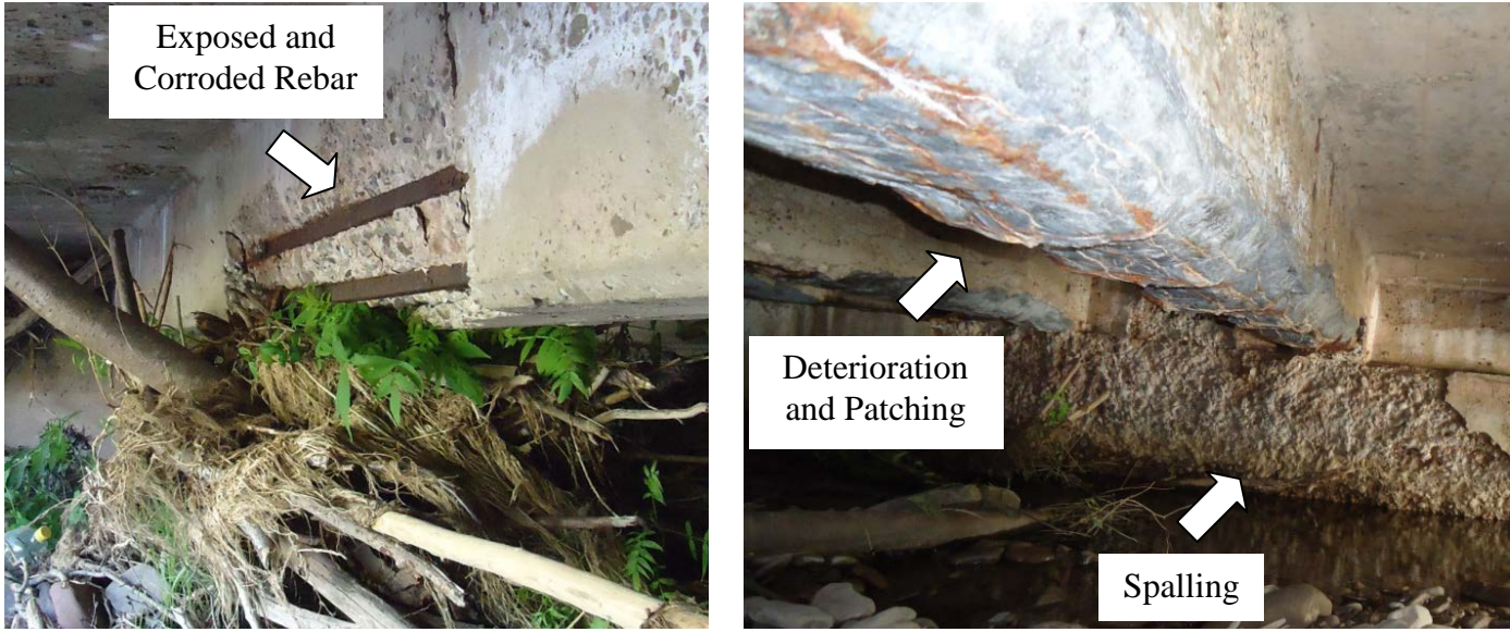
(a) Beam One Exposed and Corroded Rebar
