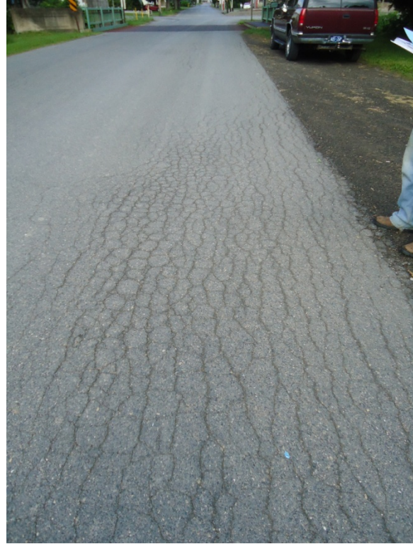
(b) Westbound Lane Edge Pavement Damage and Cracking
