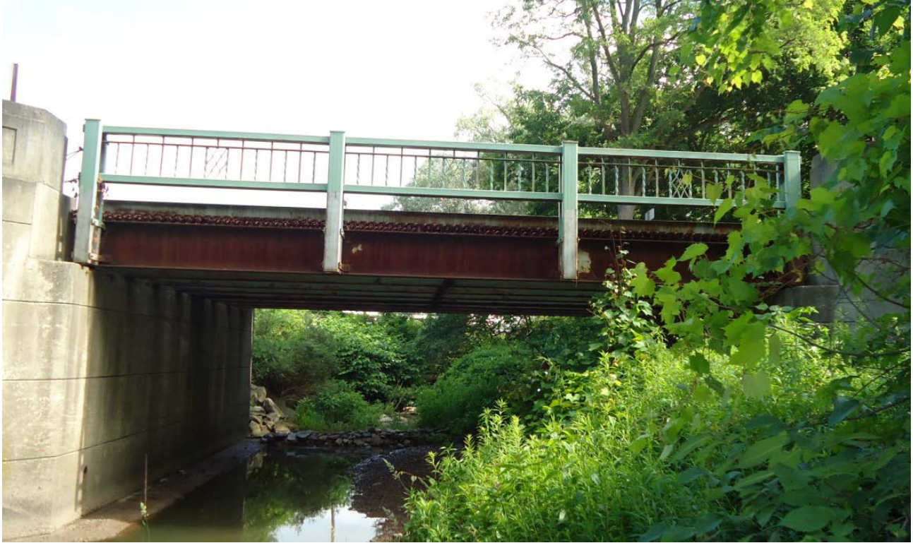
Figure 5. Bridge Two Elevation
