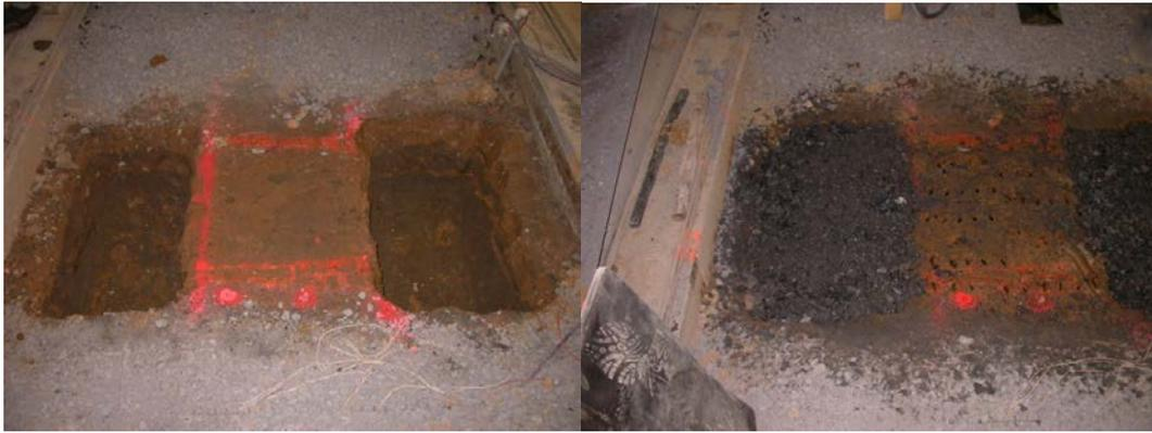
Figure 17 Test pit with soil removed and soil replaced with aggregate.
