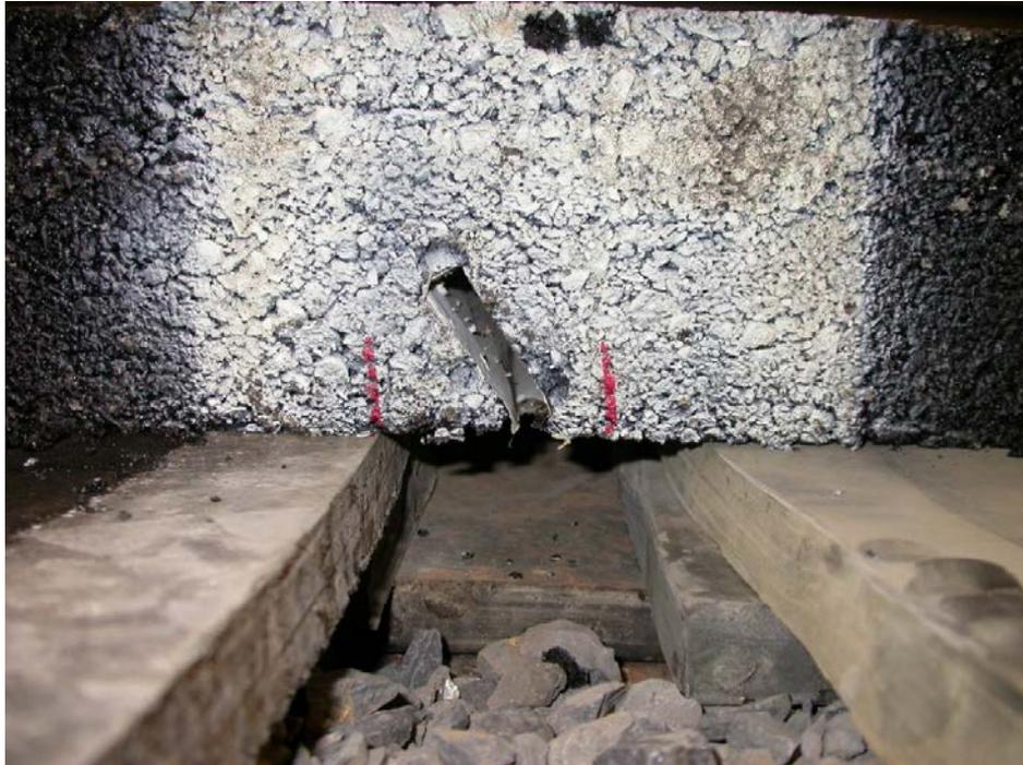
Figure 24 Photograph of the 3-inch gap under the slab.
