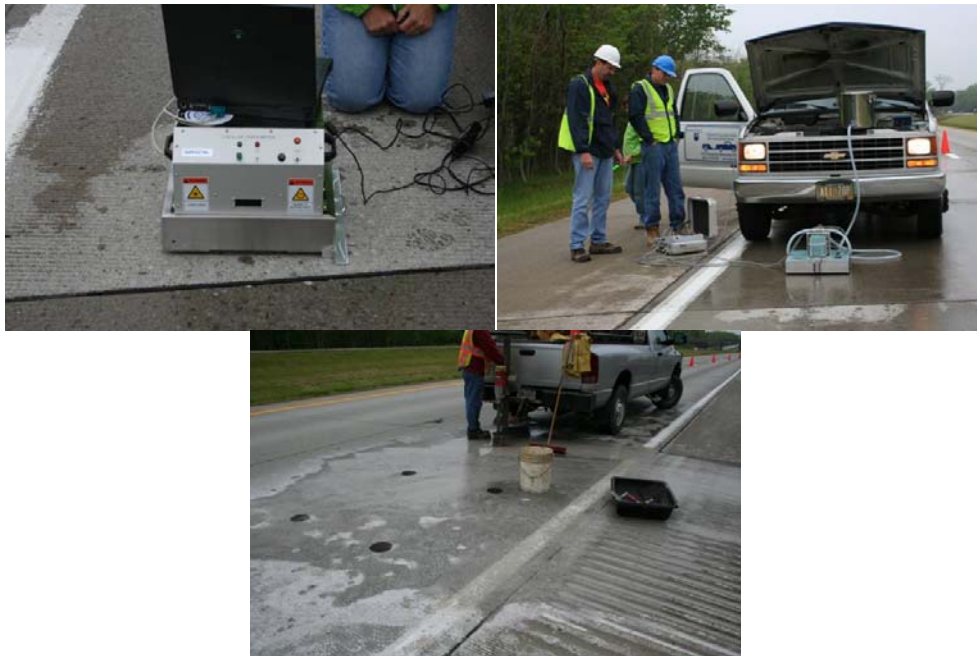
Figure 15. Onsite measurements and core drilling
