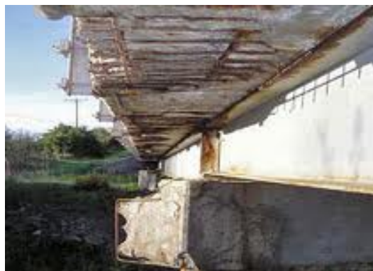
Fig. 1: Corrosion of rebar in a bridge deck overhang Source: http://www.empire-solutions.com/bridges.html
